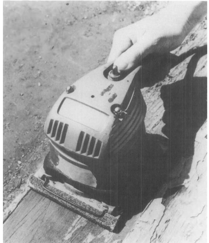
Fig. 11 The orbital sander can be used for limited paint removal, i.e., for smoothing flat surfaces after the majority of deteriorated paint has already been scraped off. Photo: Charles E. Fisher, Ill.
