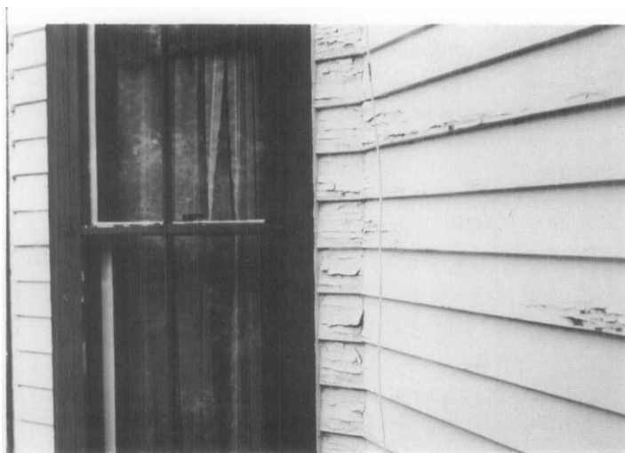
Fig. 8 Peeling to bare wood—one of the most common types of paint failure—is usually caused by an interior or exterior moisture problem. Photo: Anne E. Grimmer.
